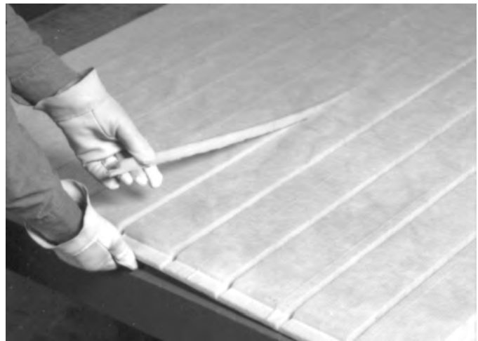
Fig. 3-34A. Removing scrap from grooved duct board.
