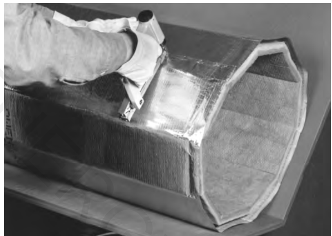
Fig. 3-34B. Stapling longitudinal joint of ten sided duct.
