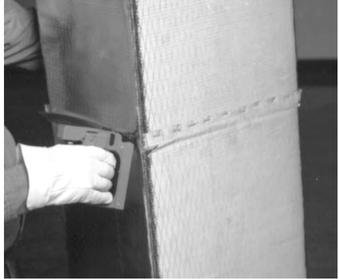
3. Staple flaps on four sided with 1/2" (minimum) outward clinching staples approximately 2" (51mm) on centers. For stapling details see Section IV, CLOSURE.
