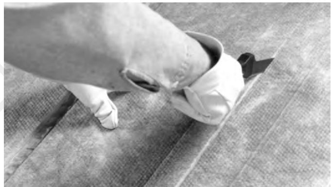
9. Using a straight knife, cut through insulation and facing along right hand cut. Peel insulation from closure flap. Board is now ready for assembly and closure to form a straight duct module.
