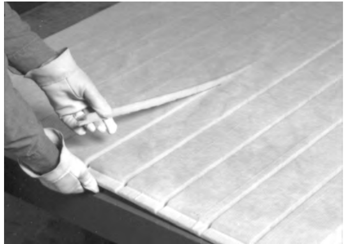
Fig. 3-34A. Removing scrap from grooved duct board.
