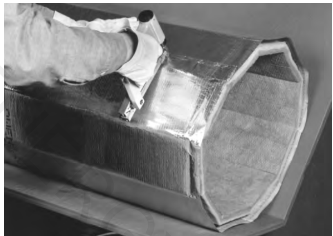
Fig. 3-34B. Stapling longitudinal joint of ten sided duct.
