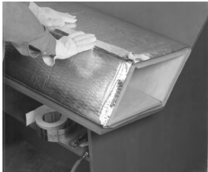
2. Fold to form the duct section, making sure ends are flush and seated properly in the shoulder of the shiplap edge.
