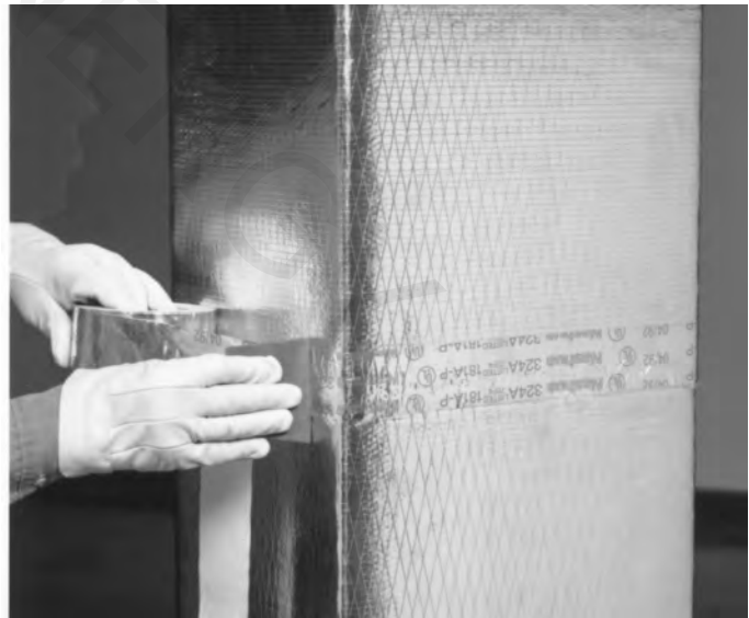
4. Complete the longitudinal seam according to procedures shown in Section IV, CLOSURE, page depending on the approved closure method chosen. (Pressure-sensitive tape shown above.) 3" tape is recommended for 1 1/2" and required for 2" board. Board must be clean and dry.
