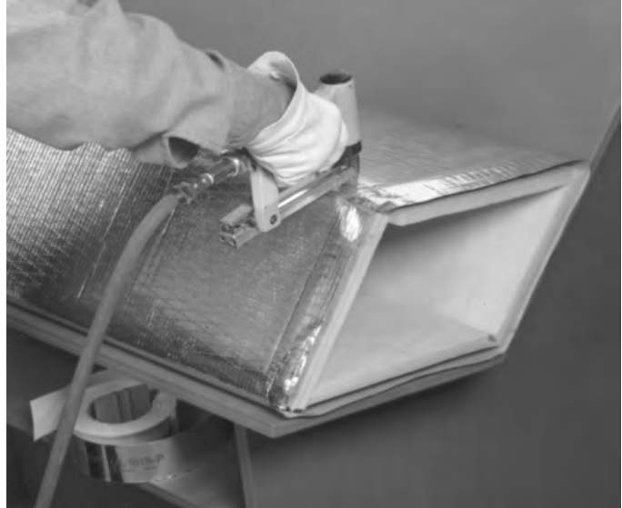
3. While holding the duct canted over at or about 30°, staple the longitudinal flap with 1/2" (minimum) outward clinching staples approximately 2" (51mm) on centers. For stapling details, see Section IV, CLOSURE.
