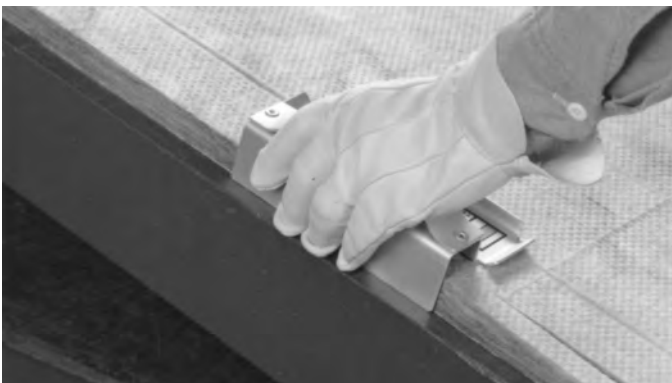
2. Cut along left edge of duct board using female shiplap tool to form shiplap edge without closure flap. Remove scrap from groove.
